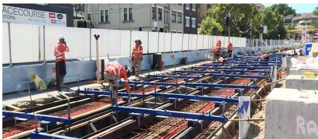
Double Track Section – rails set with positioning jigs.
