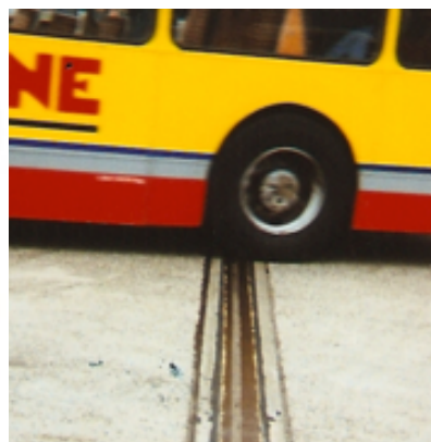
LR55 installed in a road
