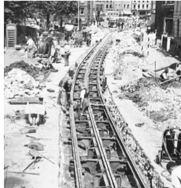
Conduit tram track construction in London
