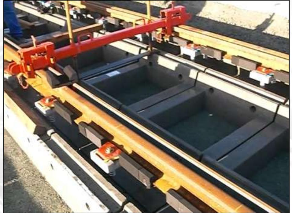
Installation of rails into precast element recess
